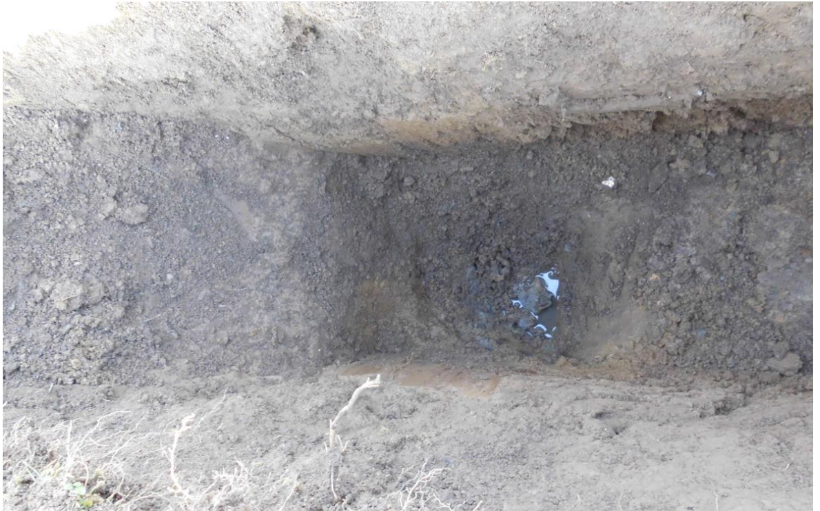
Trial Pit – Depth 0.95 – water encountered at 0.85m bgl
