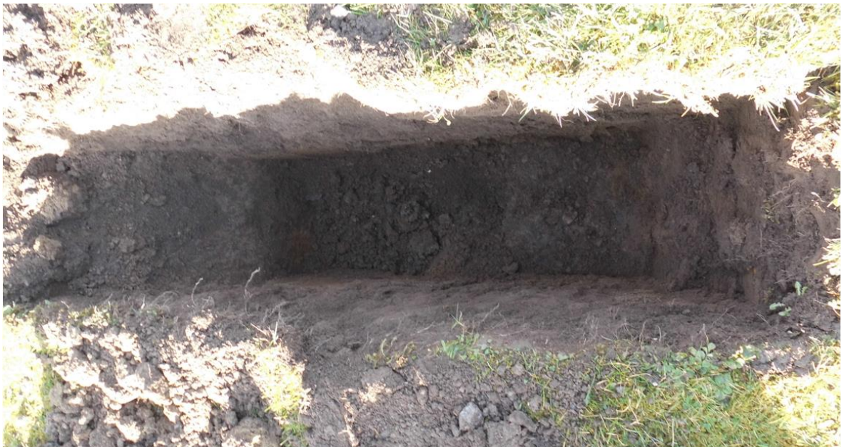
Test Pit before water added – Depth 0.75m
