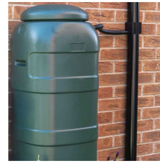
RAINWATER BUTT CONNECTION NTS
