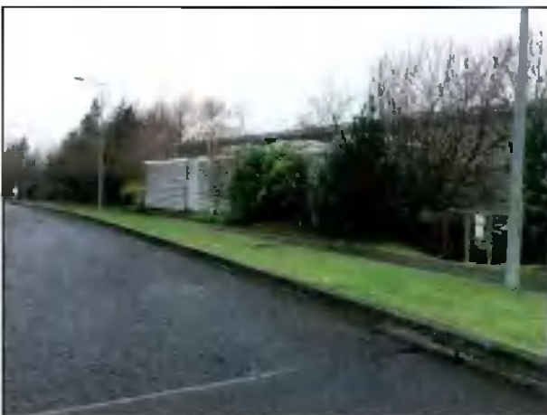
View of generator compound facing onto Orchard Avenue
