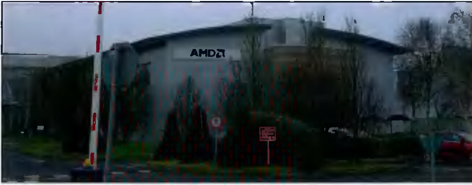
New sign on north elevation of existing facility
