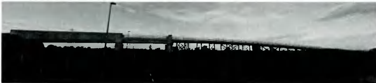
Figure 5 - View of the rail bridge and bridge ramp from Station Road looking west
