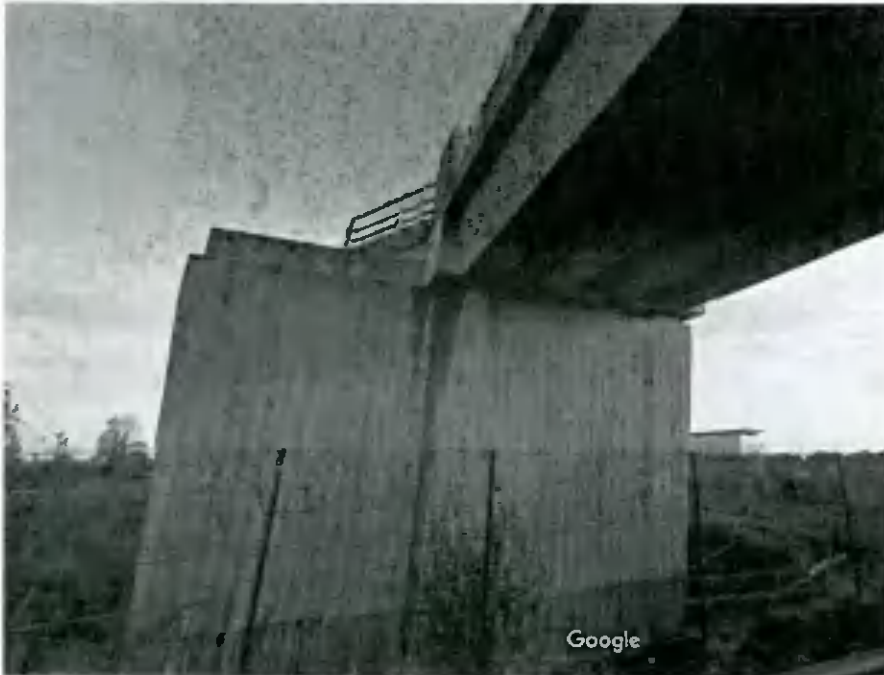
Figure 6 - Ramp support in place designed to accommodate widened ramp and bridge
