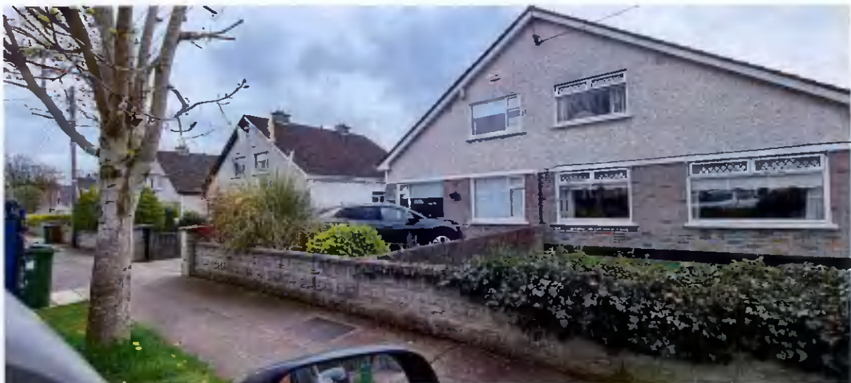
Fig 3. Site view front 13-04-2022
