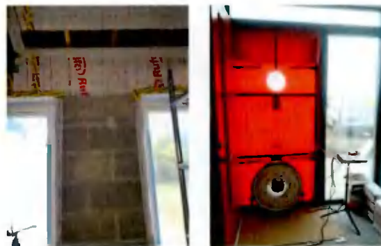
Figure 3: Air Tightness Testing Examples
