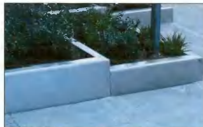
POWDER COATED STEEL PLANTER EXAMPLE IMAGE SHOWING UPPER AND LOWER TIERS OF RAISED PLANTER.
