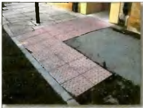
RED CONCRETE BLISTER PAVING WITH DISHED KERB TO ROAD SURFACE AS SHOWN
