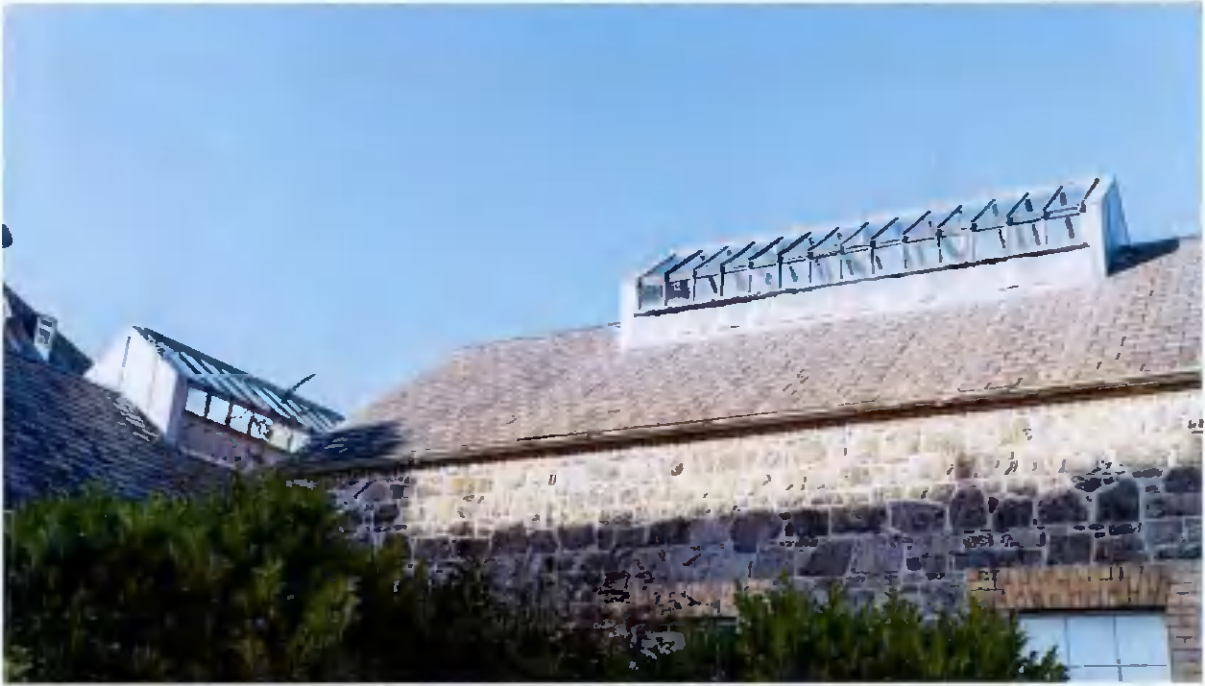
Fig. 9: Closeup Photo of Roof Lanterns
