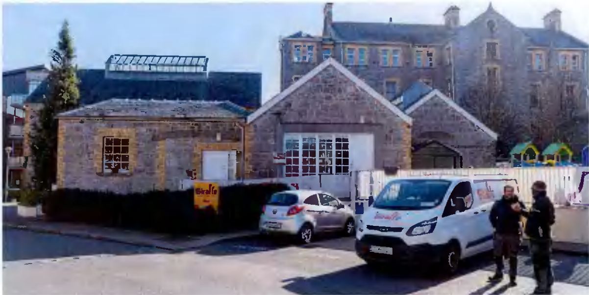
Fig. 6: Building Photo Looking West
