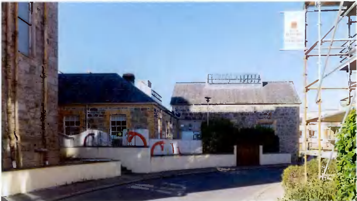
Fig. 8: Building Photo Looking South
