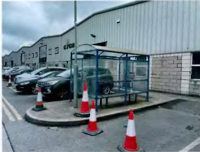
Figure 1 -- Existing Smoking structure
