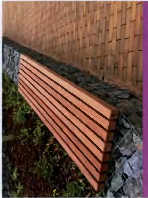
Cabion Walls With Seat
