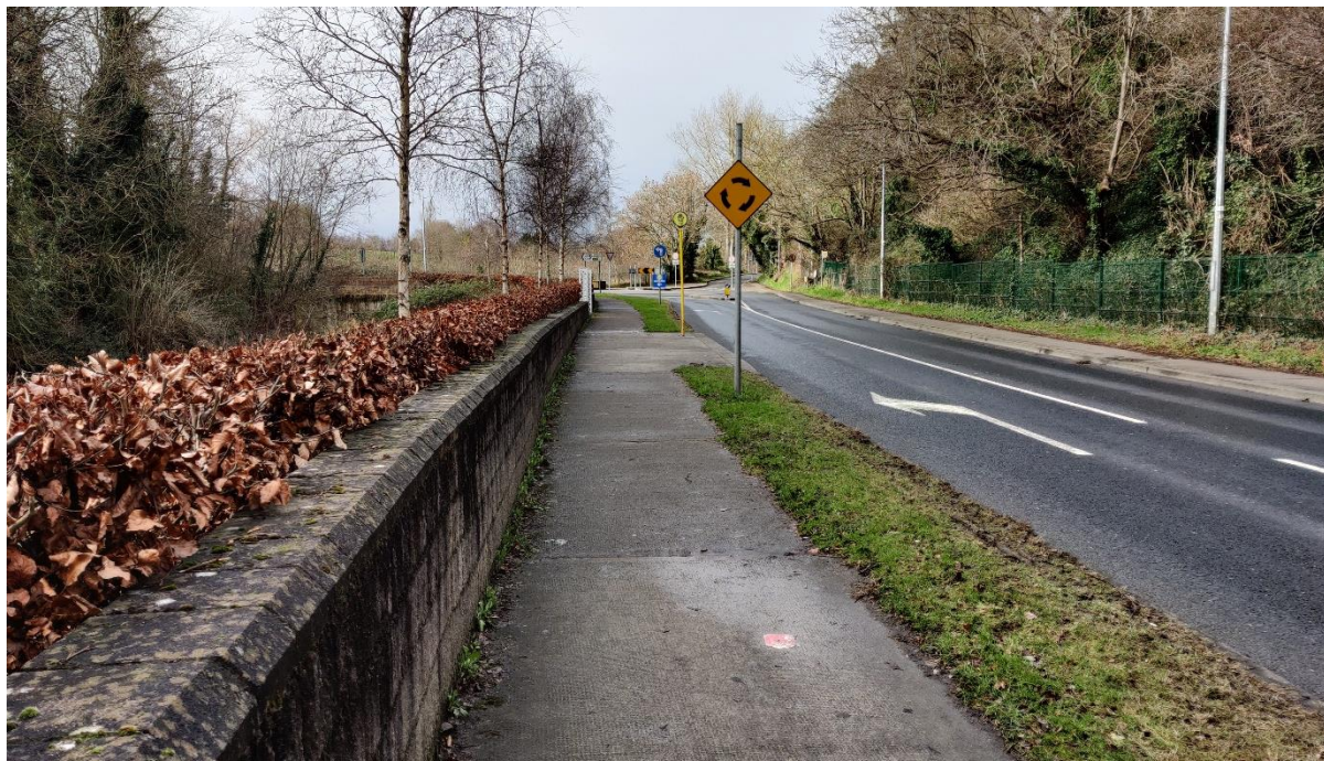
Figure 3-2: The western site section, with accompanying wall, footpath, amenity grass strip and roadway
