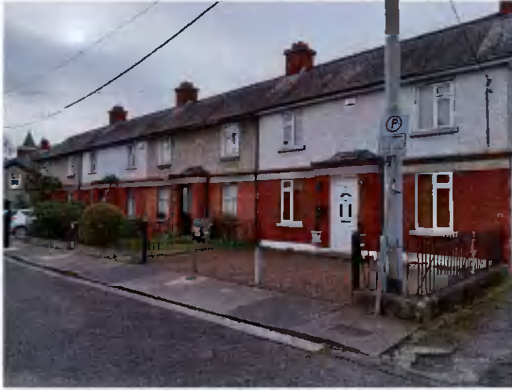
Image 04 – View of vehicular entrances to neighbouring properties
