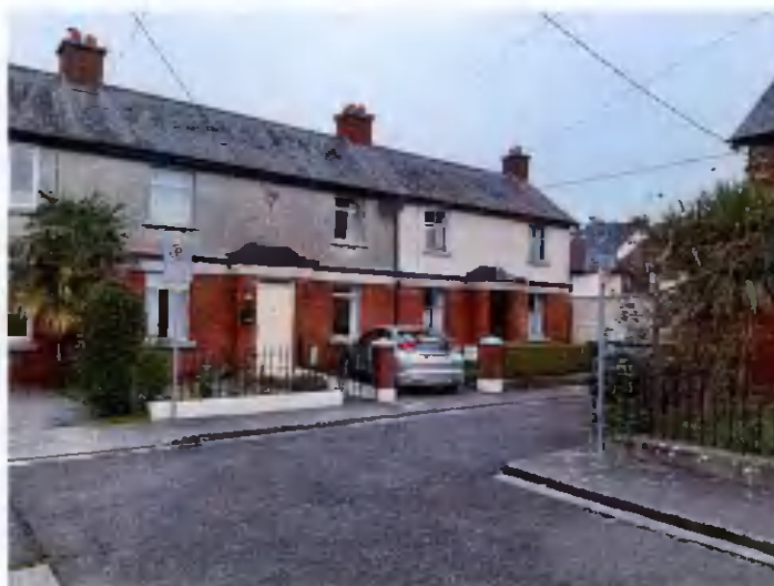
Image 03 - View of vehicular entrances to neighbouring properties
