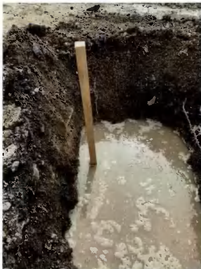
Photo No 4 Trial Hole filled with water to 750 level AT 11.42 AM
