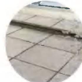
Concrete Flag Paving
