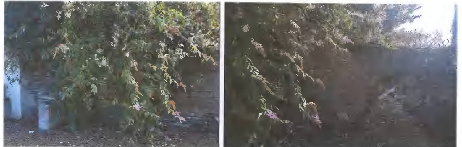
VIEWS OF THE STONE WALL FROM THE SITE - PART B NTS
