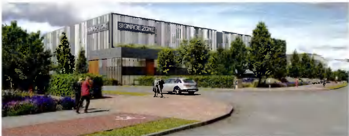
CGI View by others showing entrance from Calmount Road with subtle signage and boundary treatment, green roof. (Please note this is an Artists' Impression; planting proposals are not accurate as per the species proposed, but show an overall impression in spatial and visual terms)
