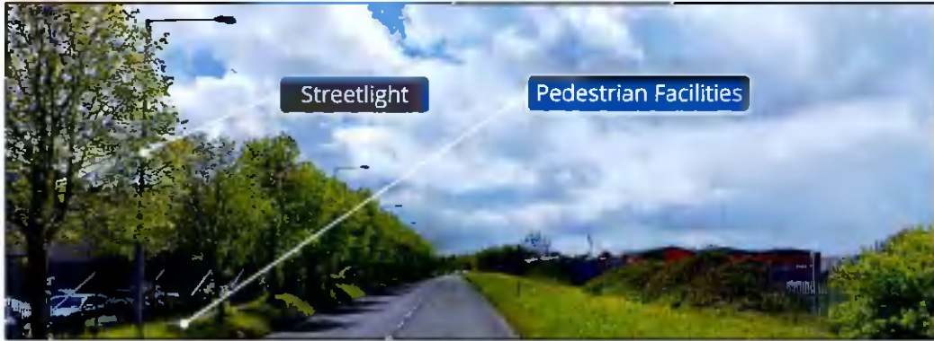
Figure 3.5: Pedestrian Facilities along Calmount Road
