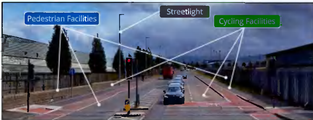
Figure 3.6: Pedestrian & Cycle Facilities on Ballymount Avenue
