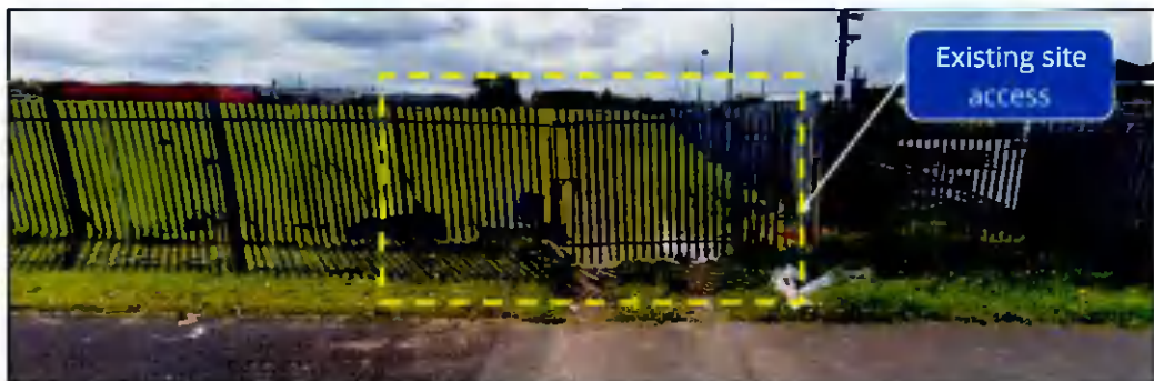
Figure 3.23: Existing Site Access on Ballymount Avenue Corridor (Source: Google Maps)
