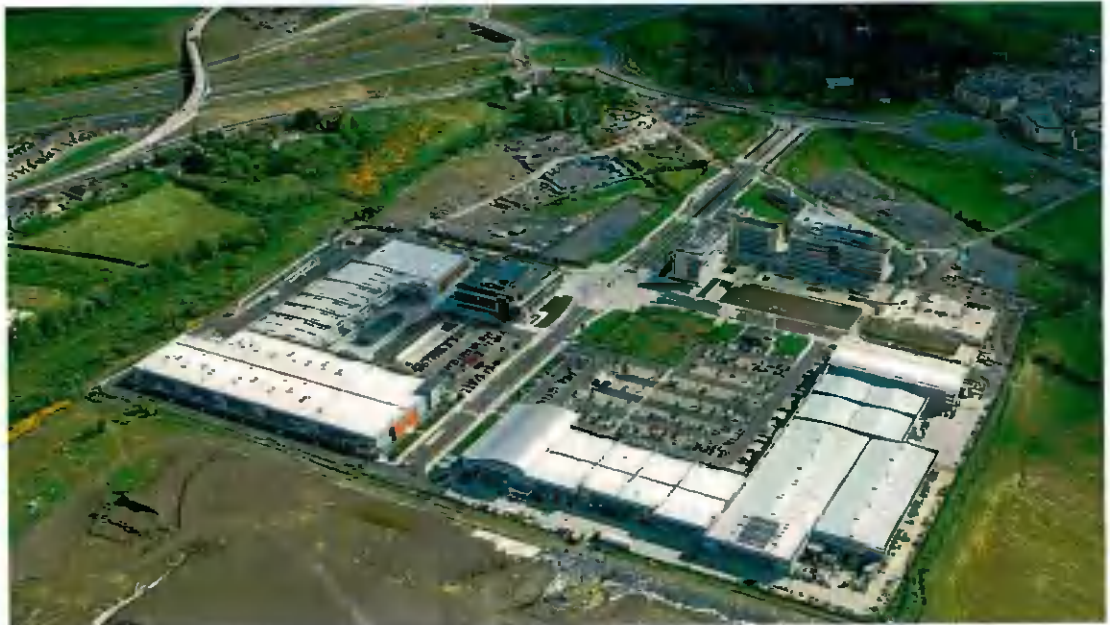
Fig 3. Aerial view of The Park, Carrickmines, Dublin 18.
