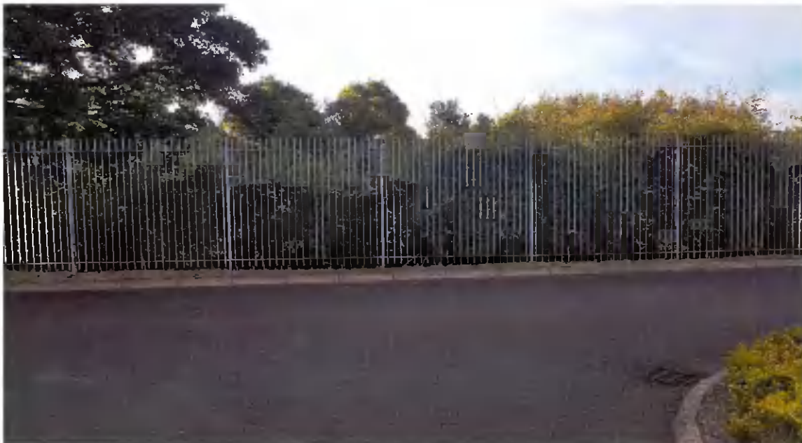
View of existing fence from Church occupied property in the area of the proposed vehicle gate.
