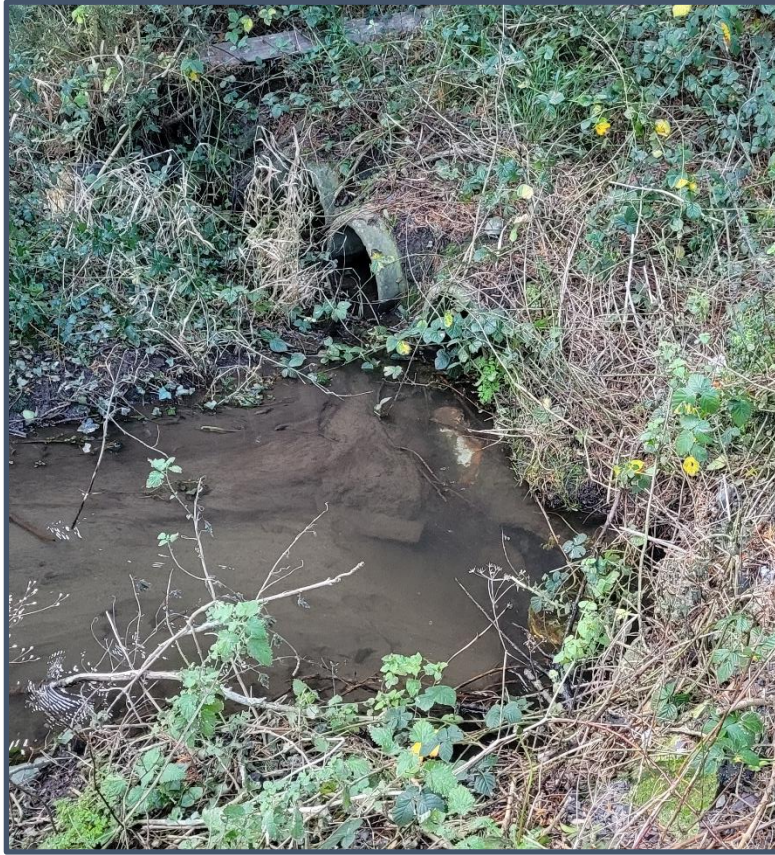
Figure 4-7 Culvert immediately downstream of Site
