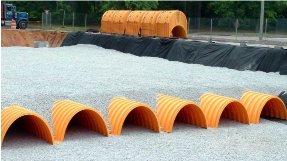
Fig.20 - StormTech Attenuation System
