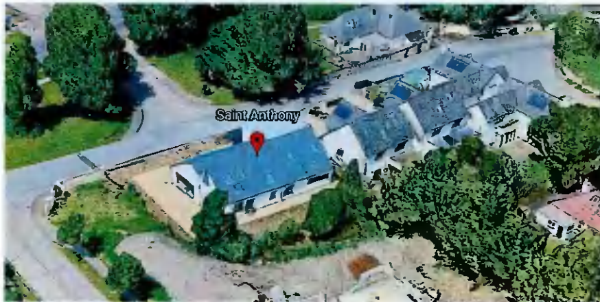
Fig. 25: The applicant site is on the tallest ground levels of this row of houses but is 4 storeys tall
