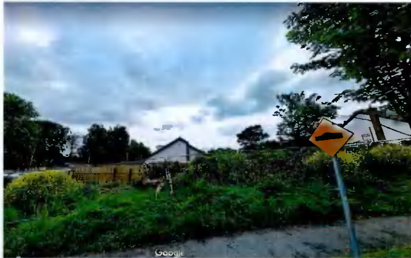
Fig. 21: The higher ground levels of the applicant site relative to client property (client's roof shown)
