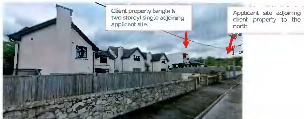
Fig. 14: The existing character and pattern of development along Old Knocklyon Road 3
