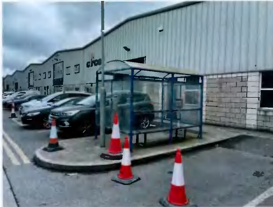
Figure 1 – Existing Smoking structure
