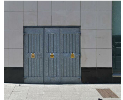
IMAGE OF INTERGRATED ESB SUBSTATION IN AN APARTMENT BLOCK
