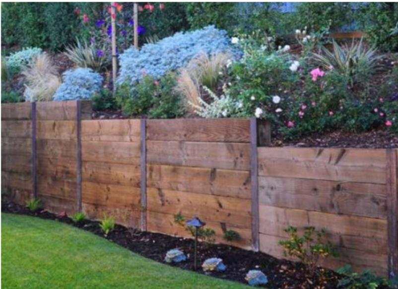
**Fig. 20 – Sample Treated Railway sleepers Slotted into RSJs.**
