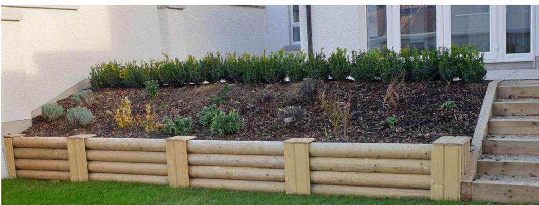
**Fig. 21 – Suggested sample showing 6 Steps allowing for a drop of 900mm**
