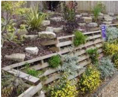
Fig. 11 – Sample Crib Wall
