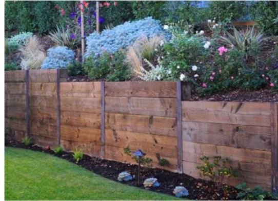
Fig. 12 – Sample Treated Railway sleepers slotted into RSJs.
