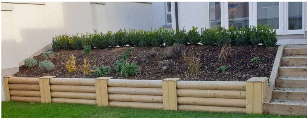
Fig. 13 –Suggested sample showing 6 Steps allowing for a drop of 900mm
