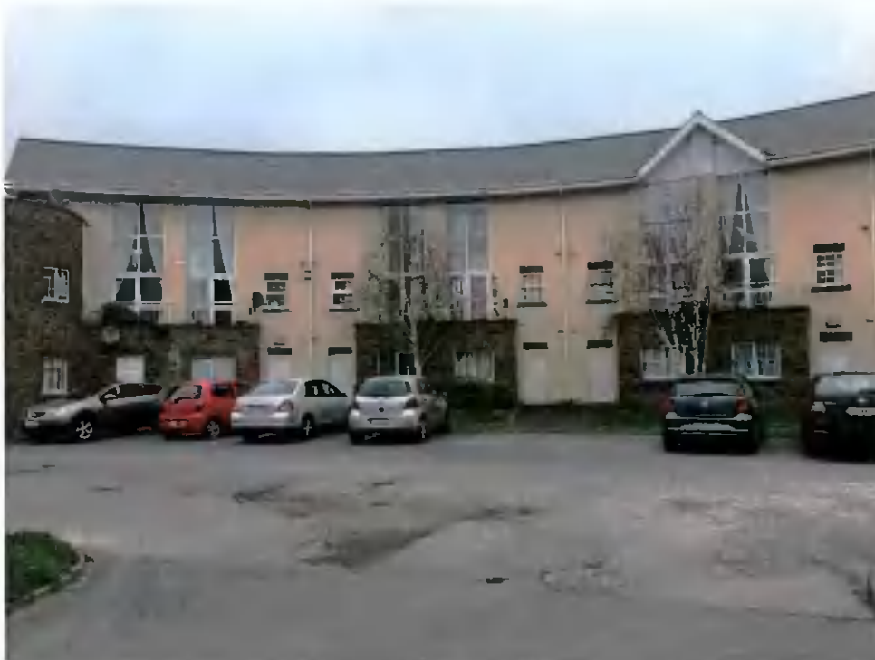
Photo 2- Showing Front Elevation of the units at The Crescent
