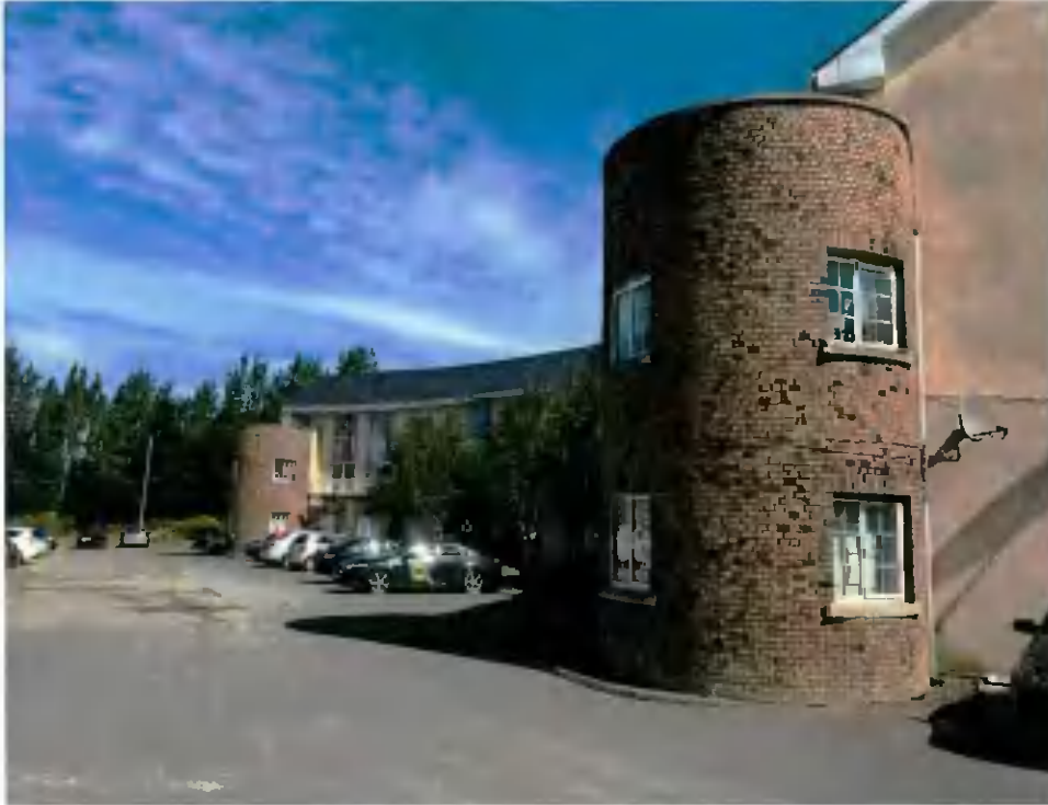
Photo 1- Front/ Side Elevation of Existing Units
