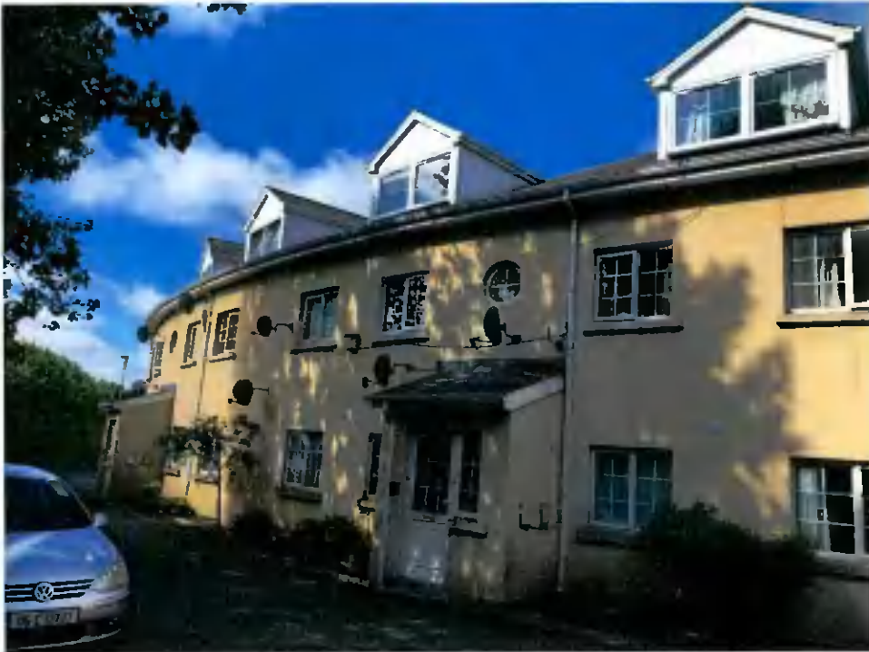
Photo 3- Showing the Rear Elevation
