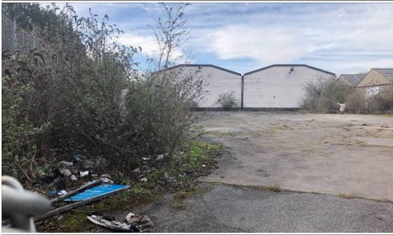
Photo 15.7: Internal view of Application Site demonstrating existing setting and condition
