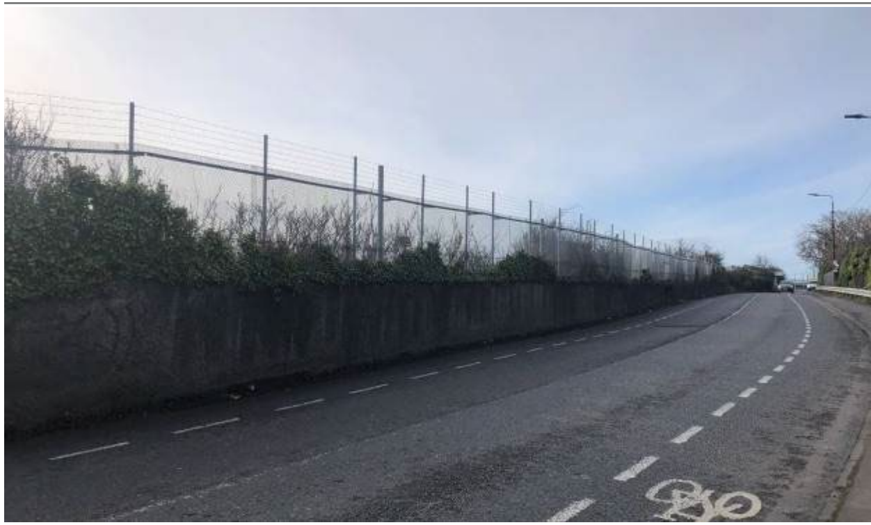
Photo 15.4: Greenhills Road on section adjacent to Application Site
