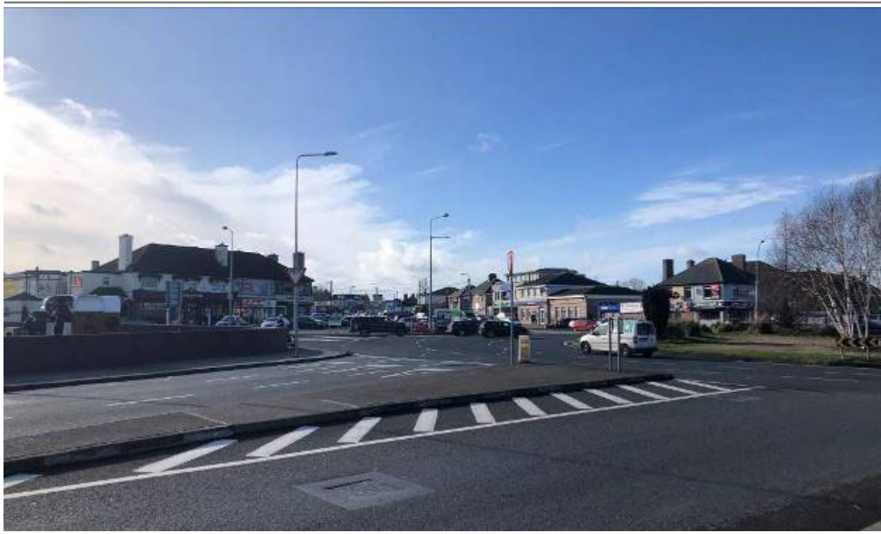
Photo 15.5: Walkinstown Roundabout looking west towards Greenhills Road and the Application Site
