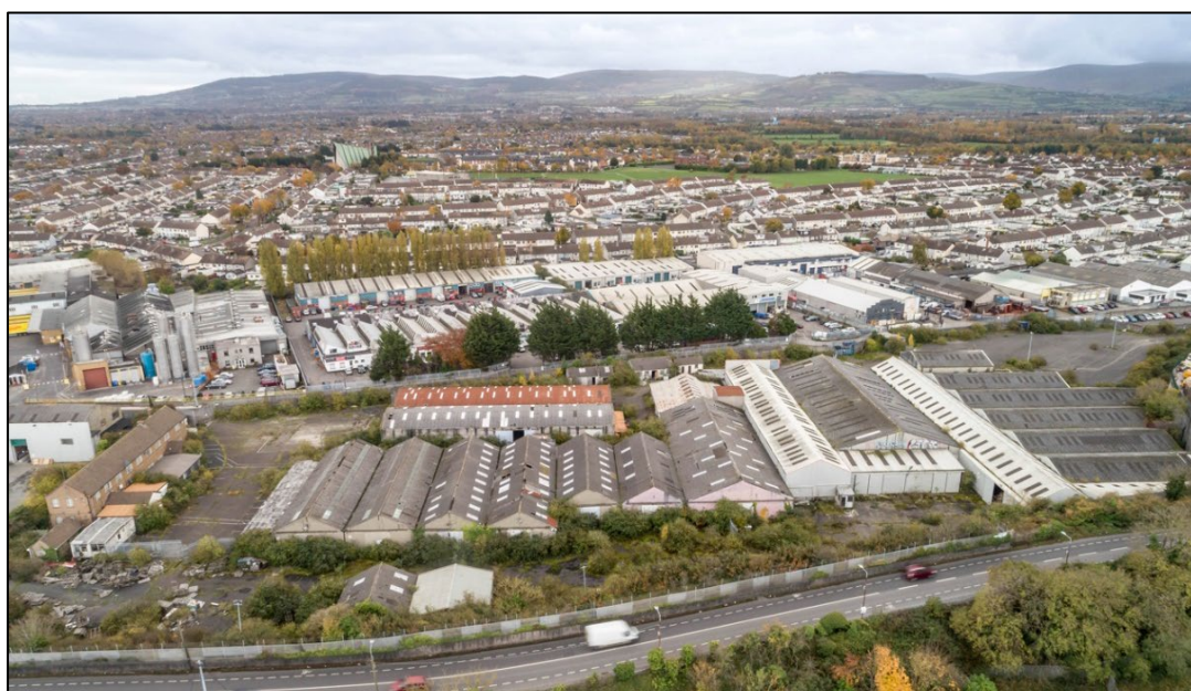
Figure 2.10 Existing Buildings on site proposed to be demolished
