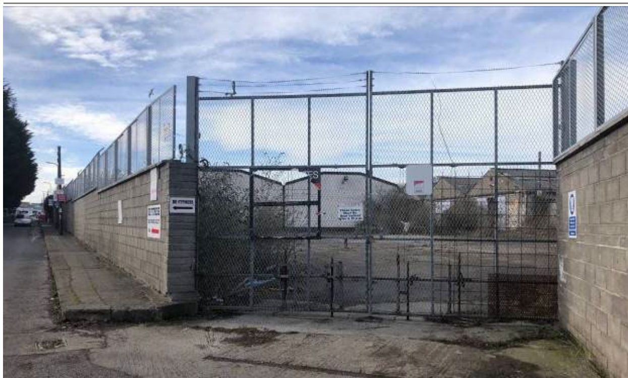
Photo 15.3: Existing Service Lane and Site Entrance to south of Application Site
