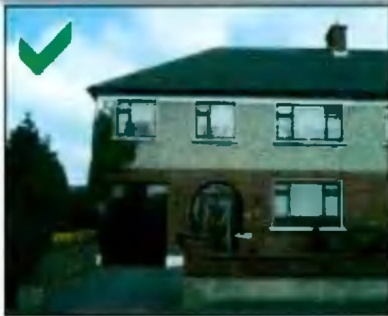
Seamless extension where materials and hipped roof match the original house
