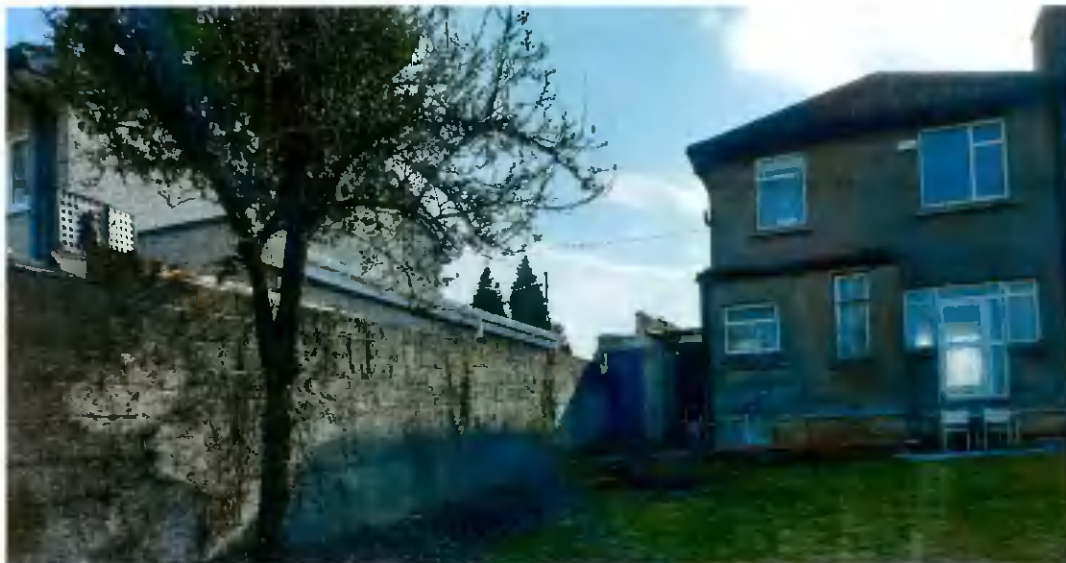
Figure 5: photograph of the north façade taken from the back garden
