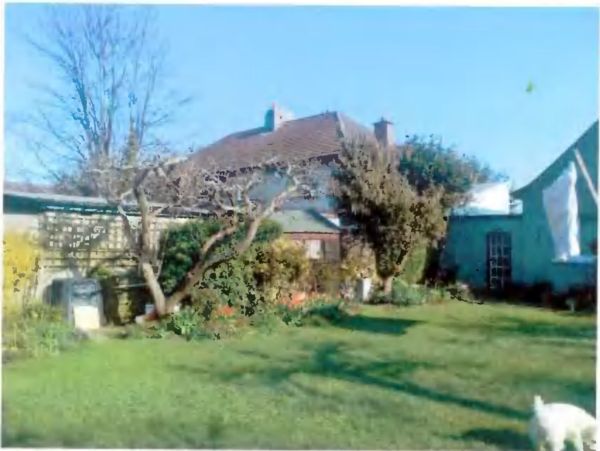
No 37, Whitehall Road Roof – Showing potential for loss of privacy from proposed dormer addition.
