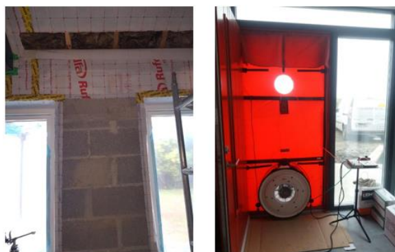
Figure 3: Air Tightness Testing Examples
