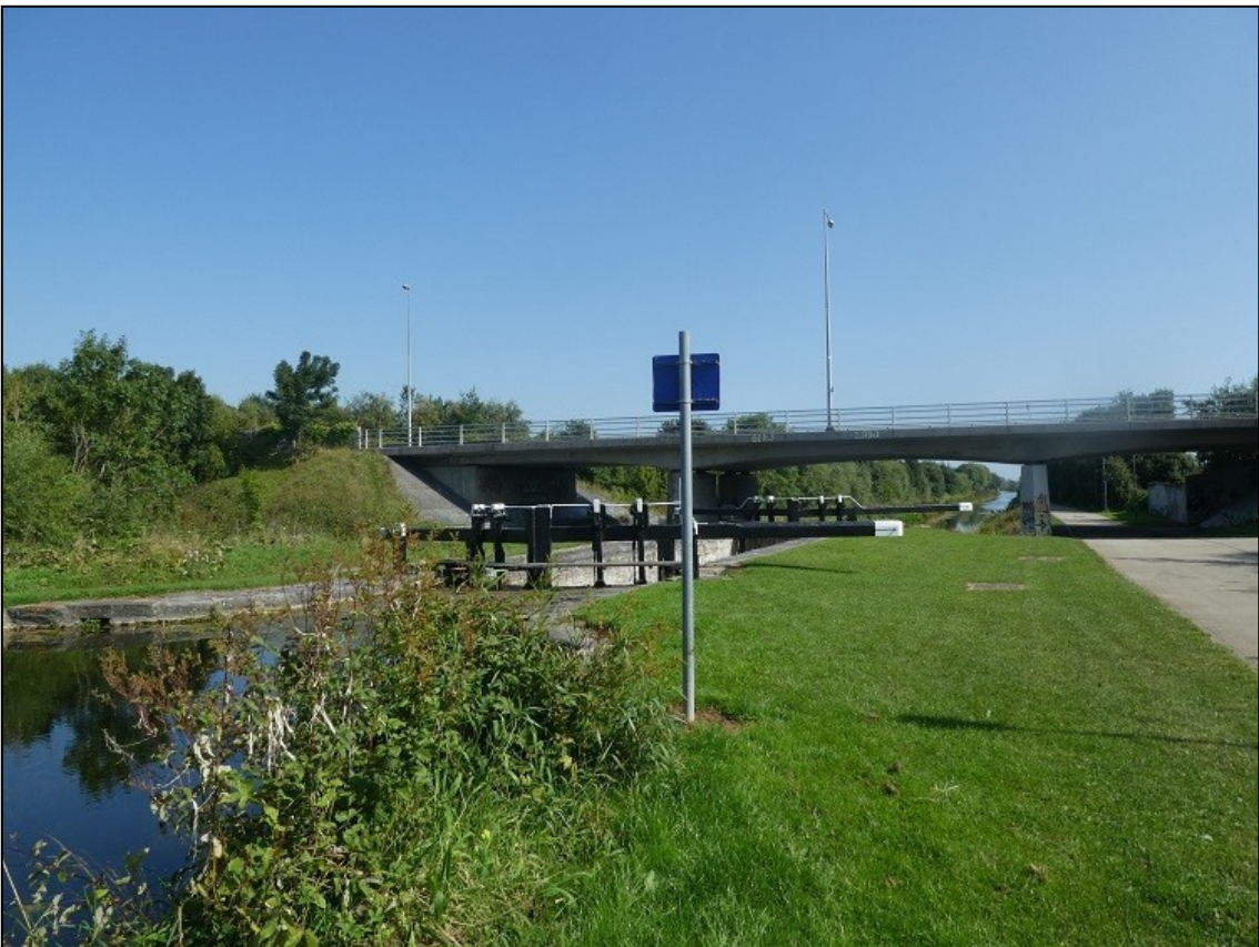
Plate 6: View of 10 th Lock of the Grand Canal to north of the subject site, facing east
