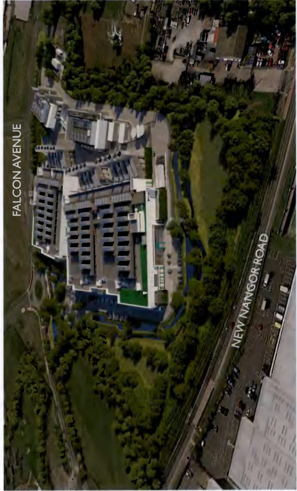
VDC Campus - Aerial View from north
