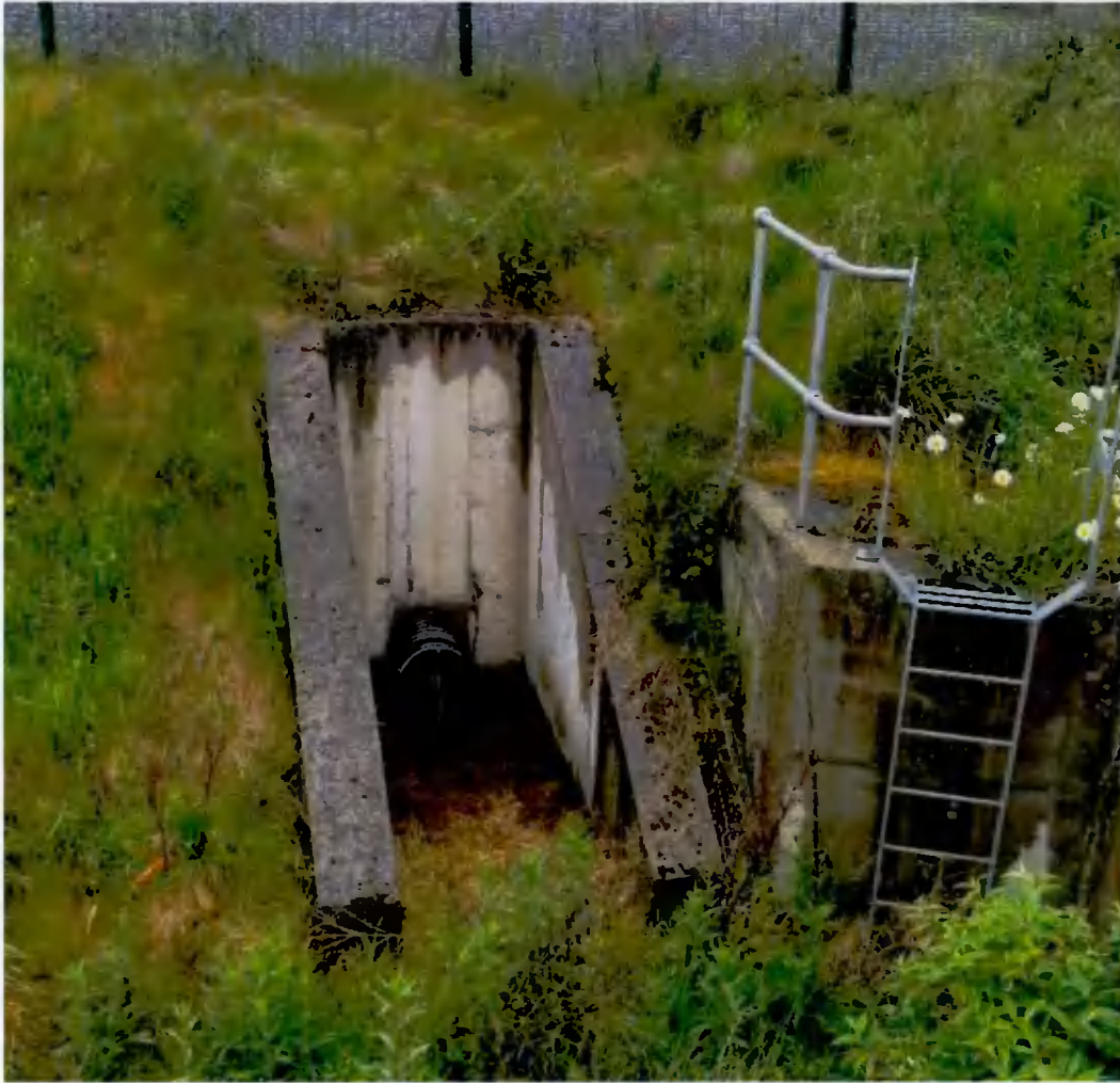
Figure 2: Surface Water Discharge Points into the channel
