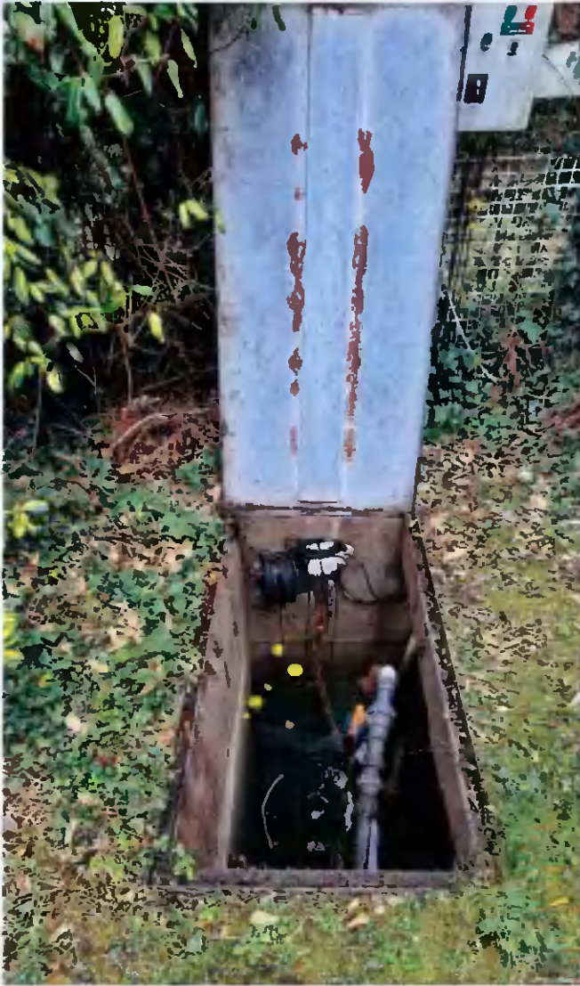
Fig 6. Existing pump chamber access manhole
