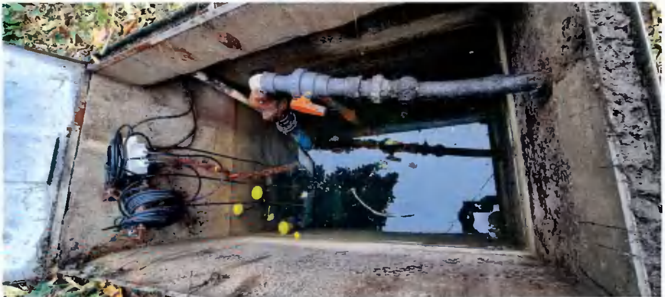
Fig 4. Existing pump chamber
