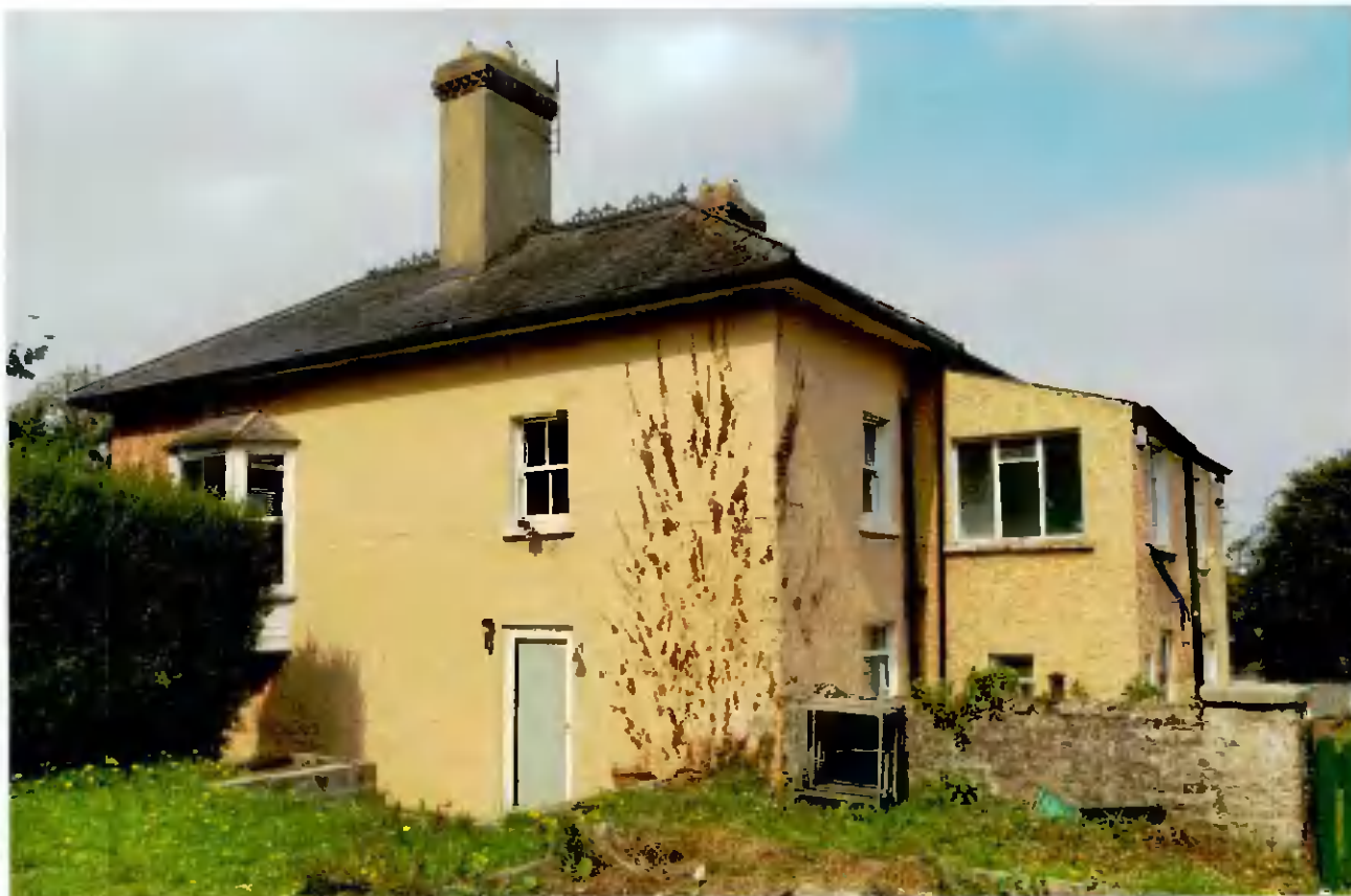
Above: Existing house as seen from the south-east
