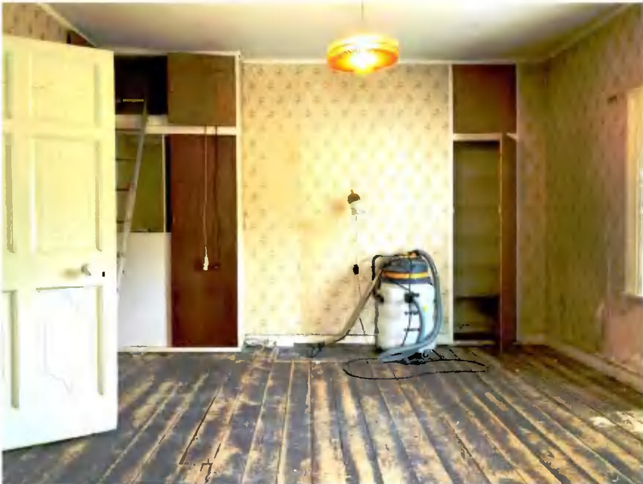
Above: proposed dining room, north-east corner of the house, note the absence of corning, picture rail and fireplace, non-original cupboards (now removed), inset into the chimney alcoves.
