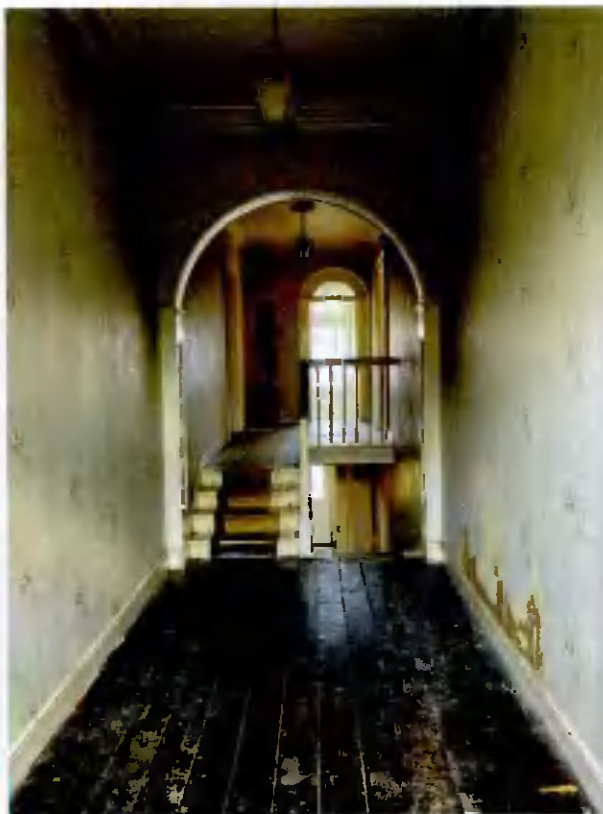
First Floor Hall: arched opening in the background
