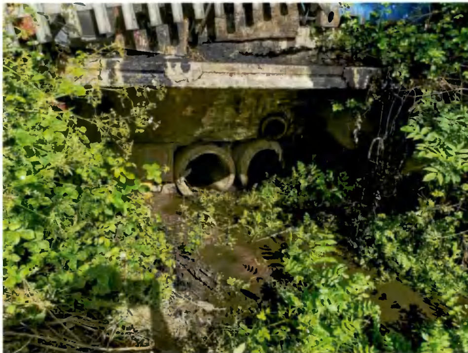
Figure 5-4 Inlet to culvert at downstream boundary
