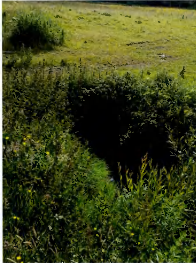
Figure 5-5 Inlet to culvert midway through the Site
