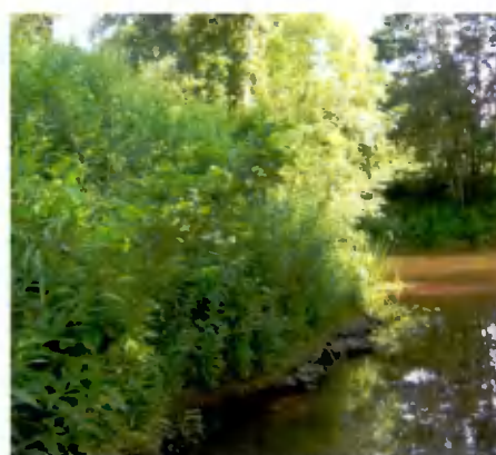
Fig 5 - Living willow wall 3 years after installation
