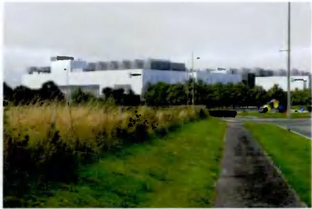
Figure 8.24: Phase 2, Year 5: Viewpoint 9 - Profile Park Road roundabout at the Site entrance looking north west
