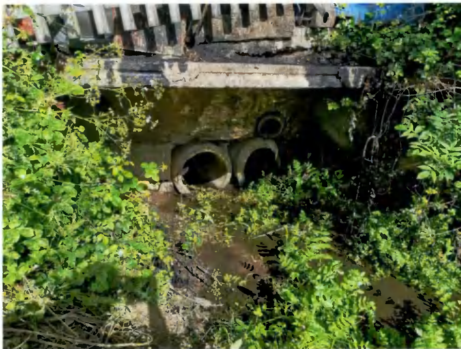
Figure 5-4 Inlet to culvert at downstream boundary
