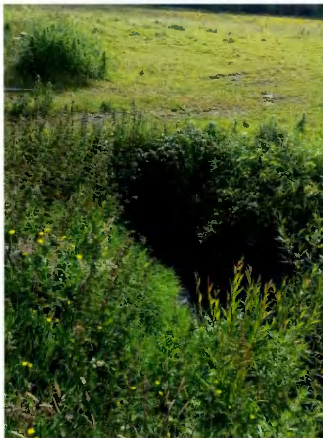
Figure 5-5 Inlet to culvert midway through the Site
