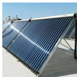
Image above showing flat plate (left) & Evacuated Tube (Right) Solar Thermal Panels
