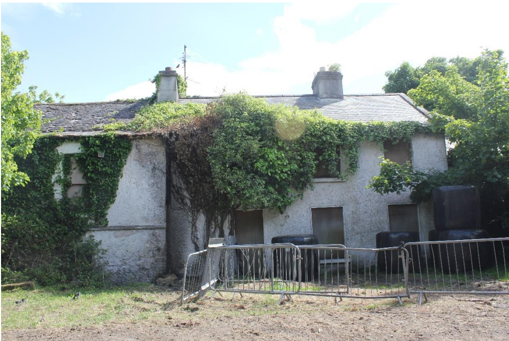
Fig. 4.6.9. View of derelict farmhouse in southern character area
