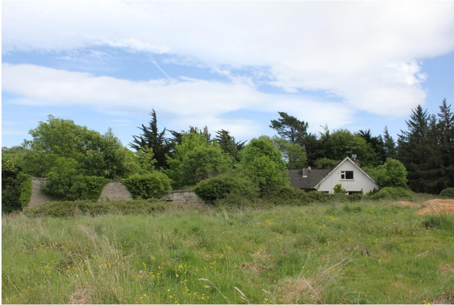
Fig 4.6.4 View of vacant and derelict residential dwelling and perimeter wall
