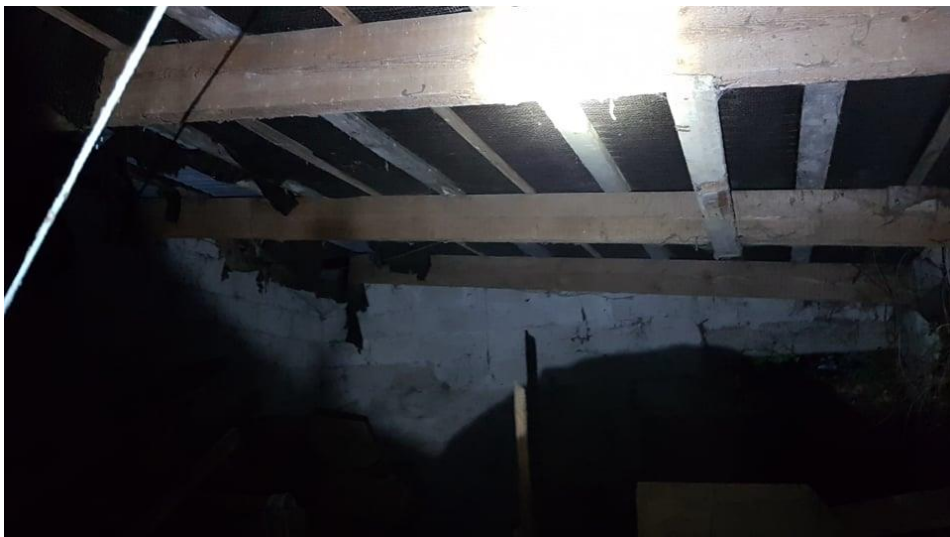
There were no signs of bats within the outbuildings
