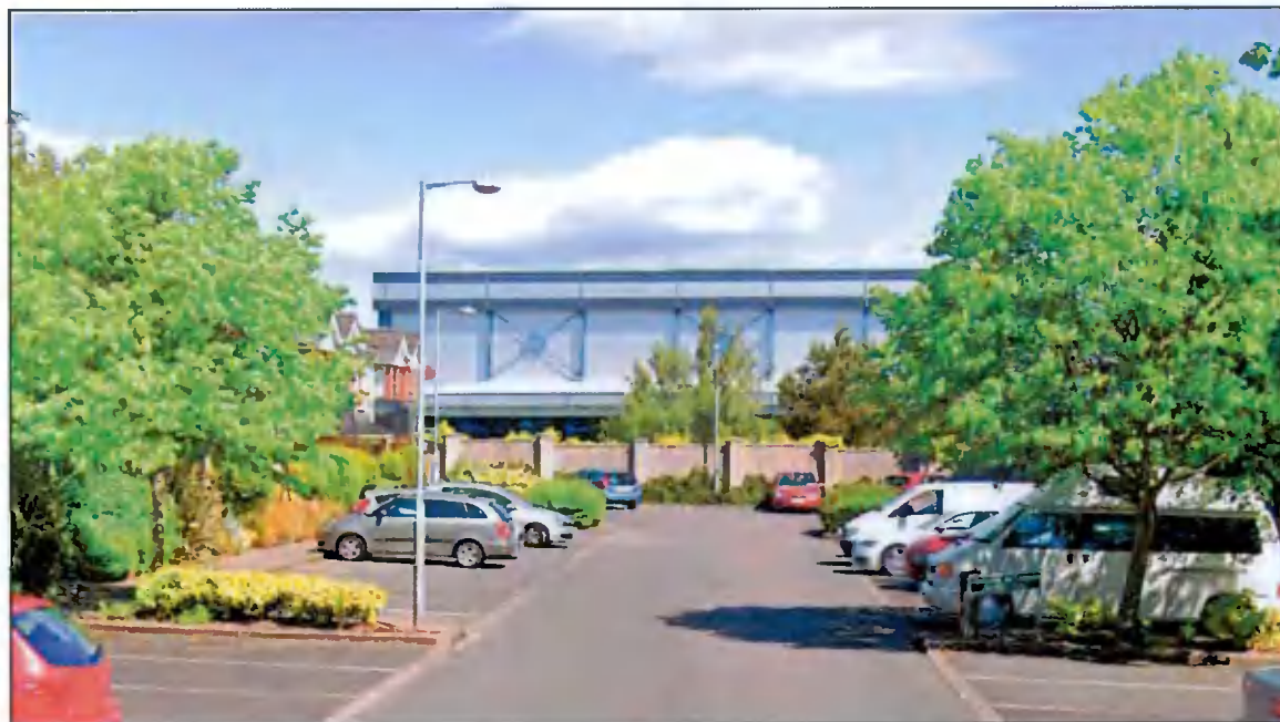
Figure 2.4: Image Showing the Milish Foods Limited Facility from the Belfry Residential Estate (Source: Google Maps, annotated by Thornton O'Connor Town Planning, 2022)
