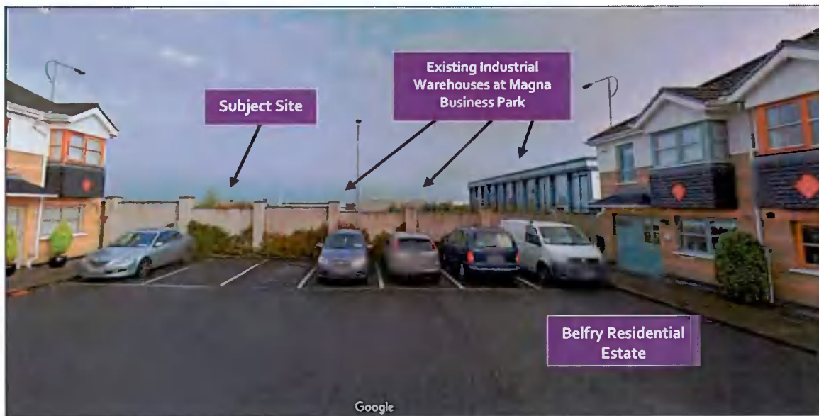
Figure 2.3: Image Showing the Location of Subject Lands from Belfry Residential Estate (Source: Google Maps, annotated by Thornton O'Connor Town Planning, 2022)
