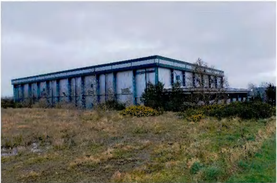
Neighbouring Warehouse development to the east of the site.
