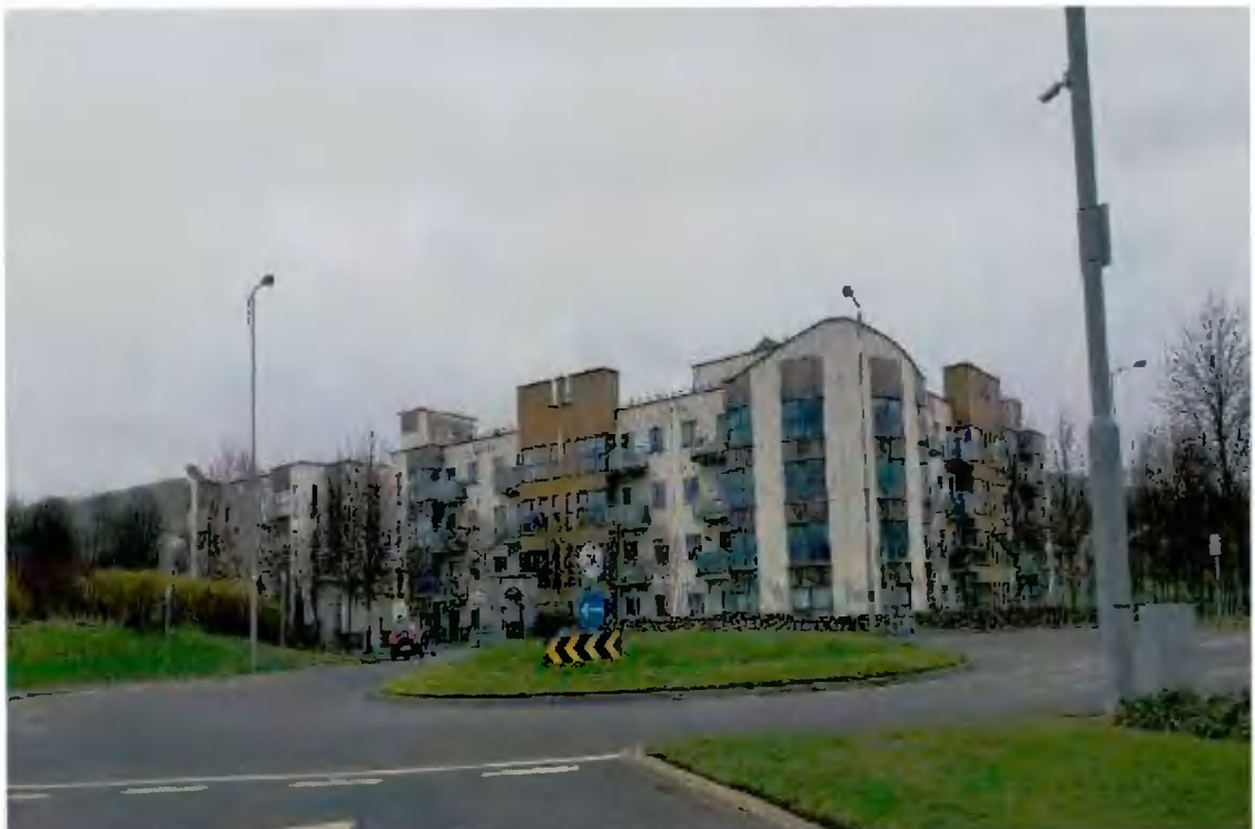
Belfry Hall to the south west of the site.
