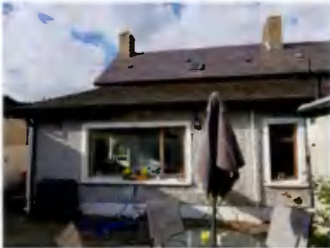
EXISTING REAR EXTENSION
