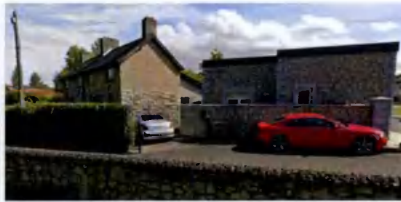
NORTH WEST ELEVATION / GABLE WALL AND NEIGHBOURING GRANITE CLAD SINGLE STORY PROPERTY, 1 ODIN'S WAY
