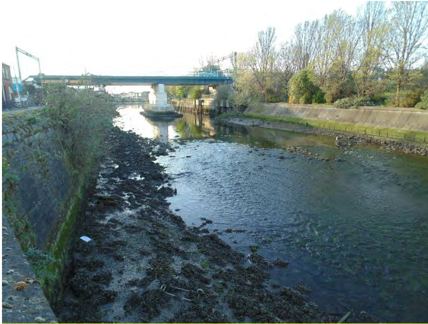
Plate 3.7 The River Tolka in the lower tidal reaches showing modification and retaining quay walls
