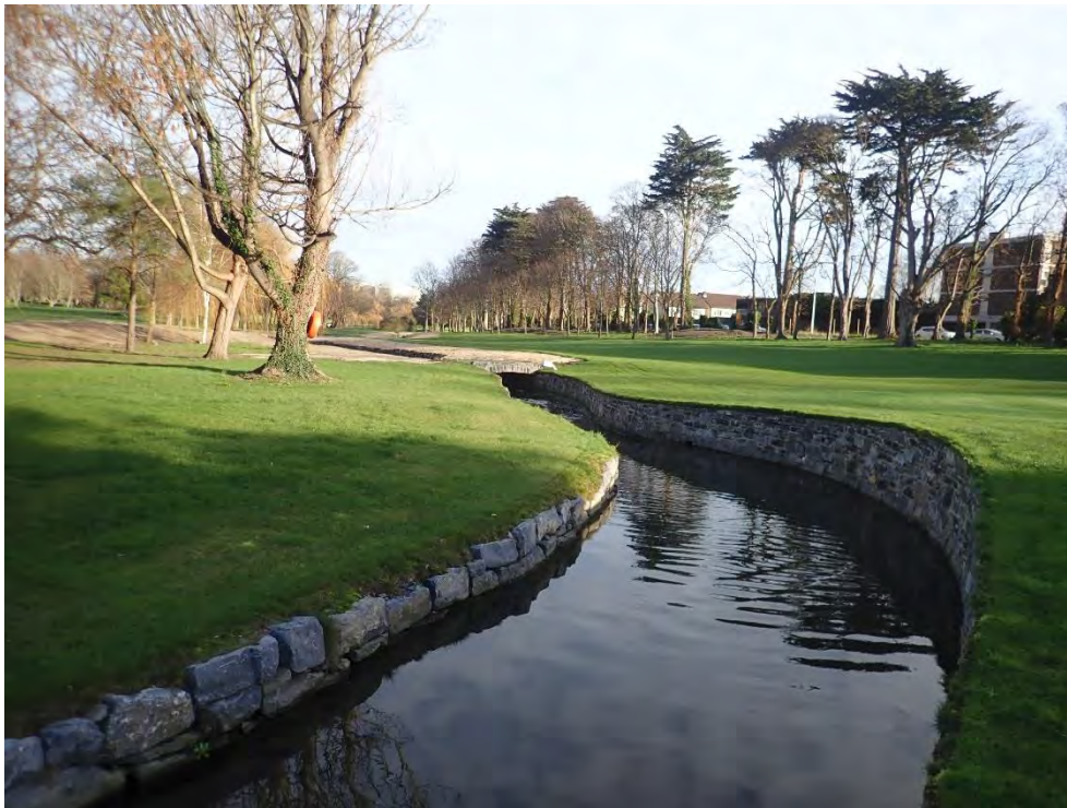
Plate 3.22 The Elm Park Stream flowing through Elm Park Golf and Sports club
