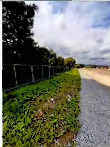
View from Existing Work Site along Proposed Site Boundary
