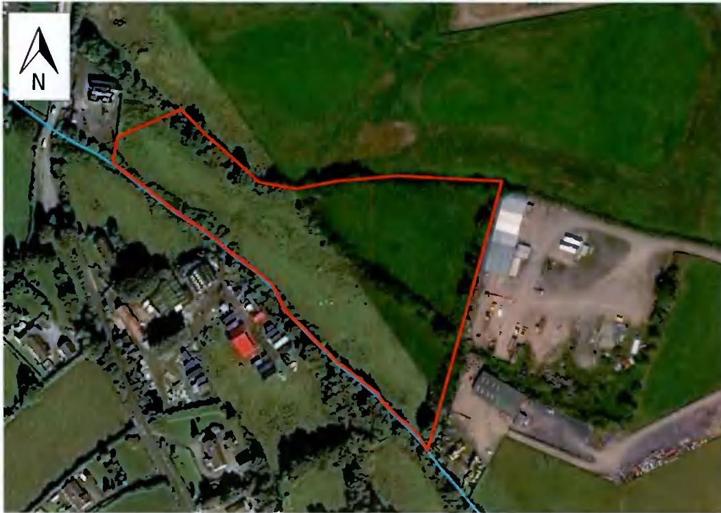
Plate 1. Aerial view of proposed infill site.
