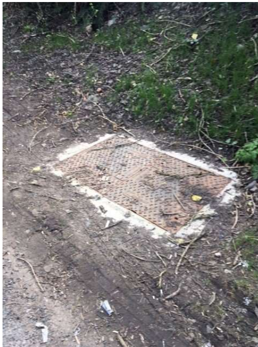
FIGURE 4. NEWLY INSTALLED CHAMBER.
