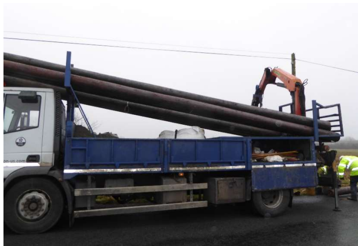
FIGURE 2. UTILITY TRUCK CARRYING UTILITY POLES AND TRUCK MOUNTED AUGER
