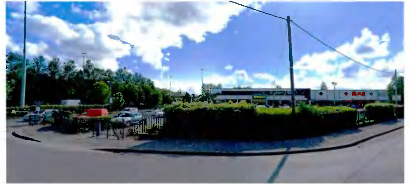
West South West View
